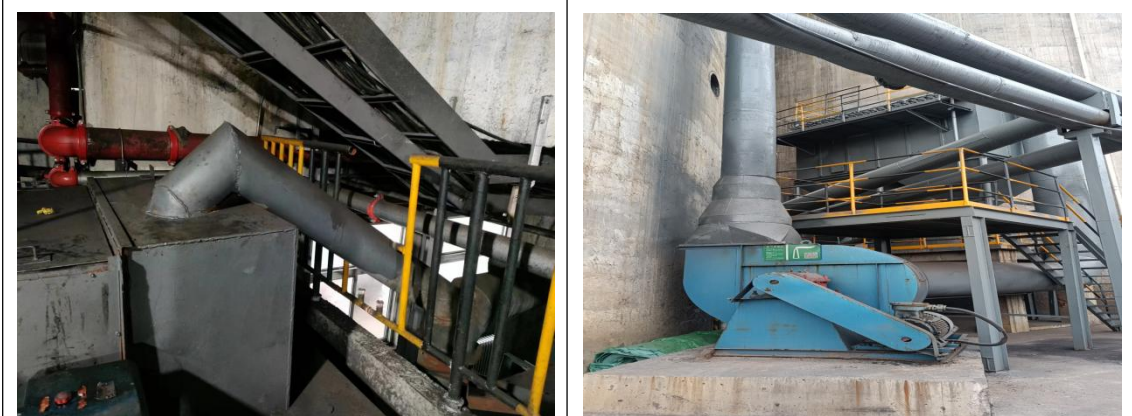
贮配煤筒仓 2#仓下系统废气
